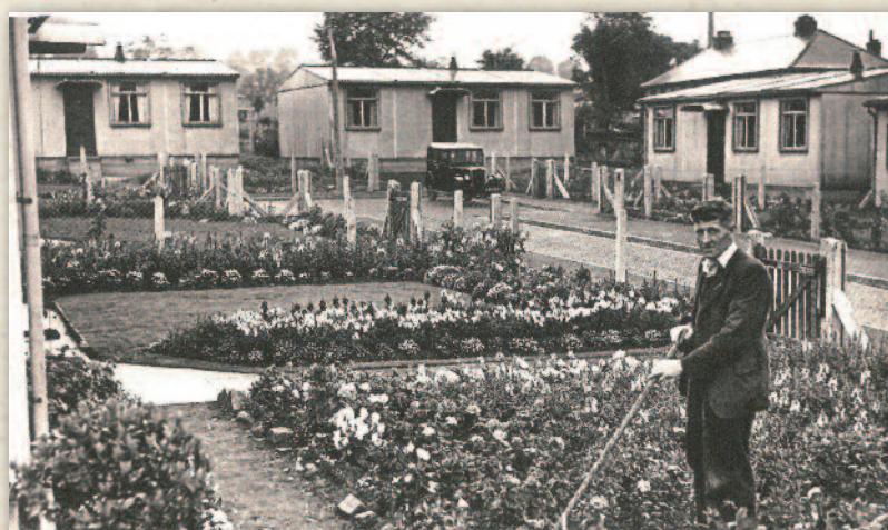
Weston Drive Prefabs 1953
